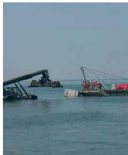
Recovery Operation using the RTCH
